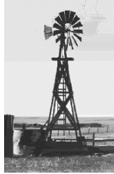
A steel-bladed water pumping windmill in the American Midwest (late 1800s)
